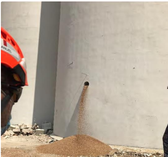
Figure 3. Test hole (25 cm diameter)
